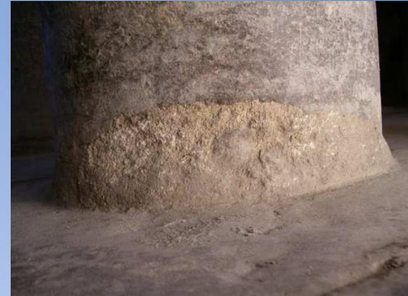
Decay caused by capillary rising damp
