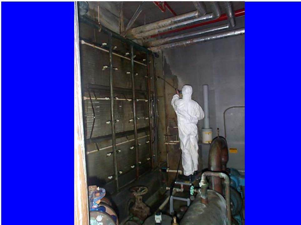
**Figure 2: Cleaning of the humidifiers**
