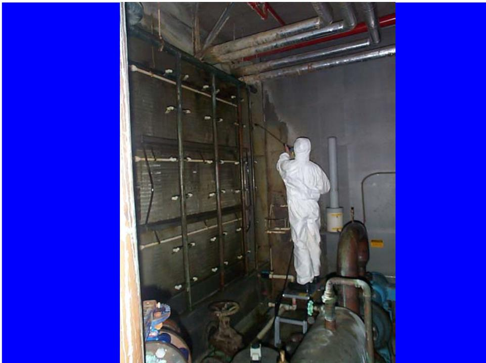
**Figure 2: Cleaning of the humidifiers**
