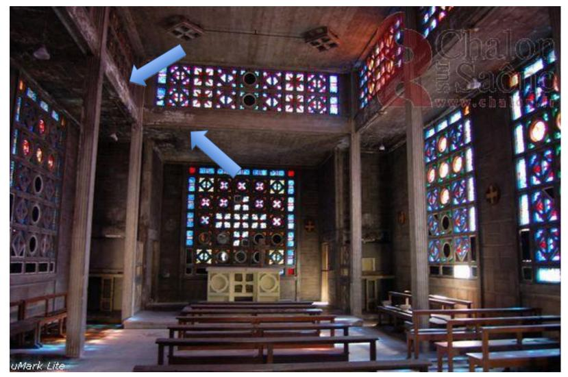
Chappelle de la Colombière – Water percolating inside the concrete envelope, pinpointed by efflorescence. Potential risk of damaged structures for thenardite-mirabilite cycles. Hypothesis to be verified.
