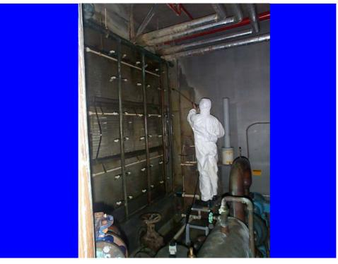
Figure 2: Cleaning of the humidifiers
